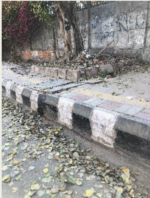
Onsite Missing Edge Line
