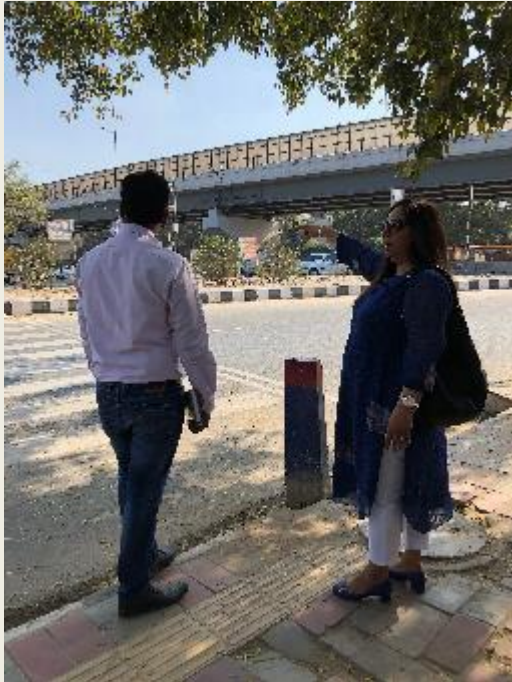
Onsite issue of missing kerb cut
