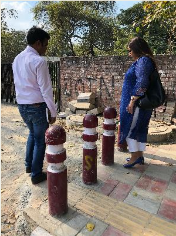
Onsite incorrect placement of Bollards
